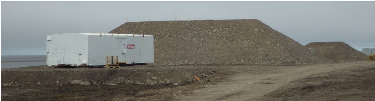
Figure 3-4 Surface Explosive Magazines and Berms
