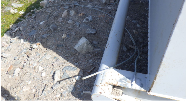
Figure 3-5 Surface Explosive Magazines – Grounding
