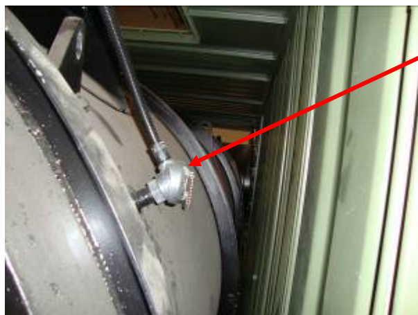
2. Two Secondary Thermocouples on Secondary Chamber body and beside the burner
