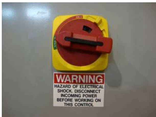
Power is OFF in this position
