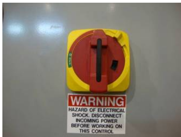
Power is ON in this position
