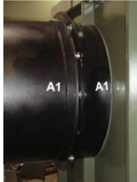
Correctly Installed Breech on Primary Chamber
