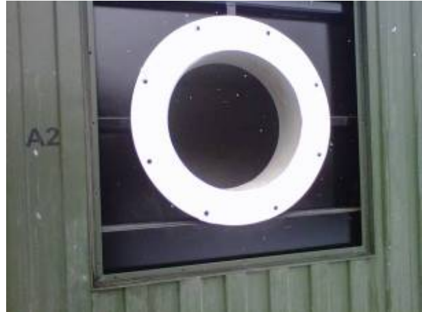
Correctly Installed Gasket
