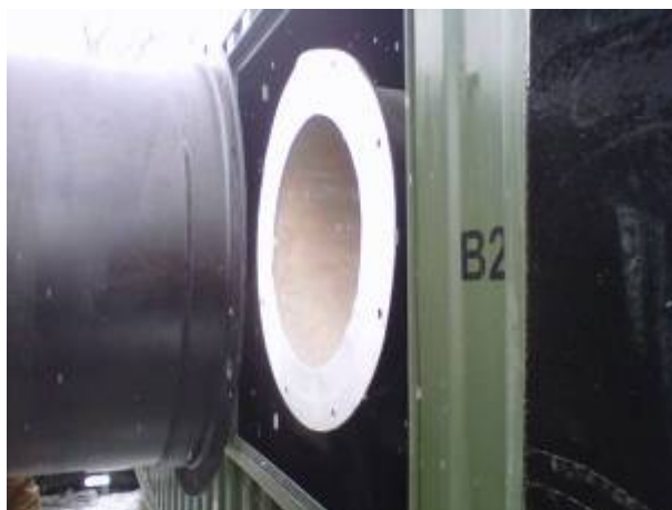
Correctly Installed Gasket
