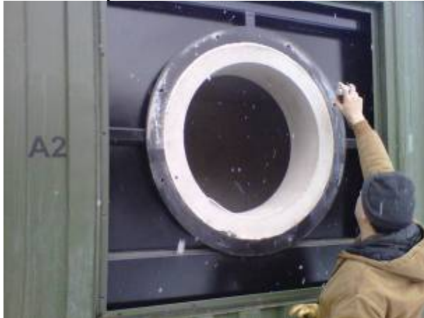
Gasket adhesive spray being applied
