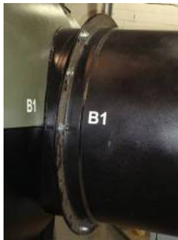
Correctly installed Breach on Secondary Chamber
