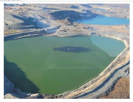
Figure 2-5: Aerial photograph of Goose Pit during initial operation in August 2024 of Diffuser/Raft 1 showing upswelling of dark hypolimnetic water into green surface waters around the aerator raft.
