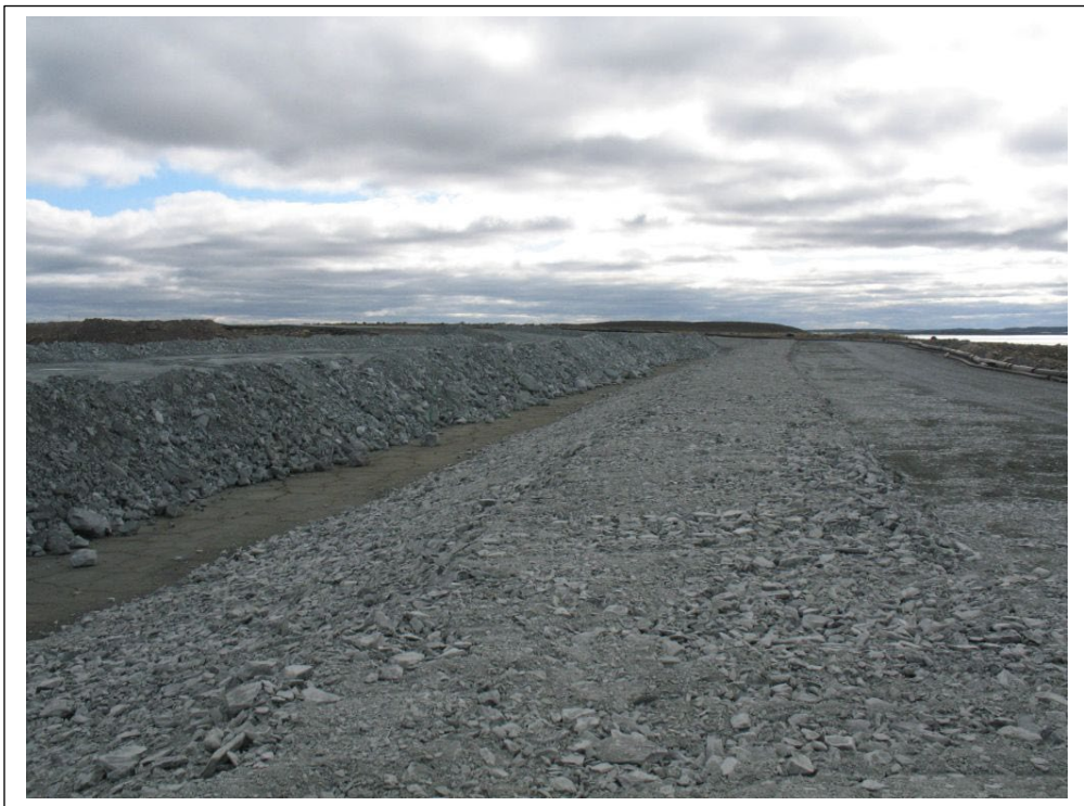
Photo #16 SD 1, new rockfill cover over liner
