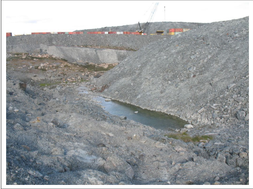
Photo#27 South Camp Dike. Downstream pool retained by waste rock pile
