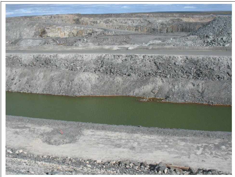
Photo #21 Pond at Central Dike. West Road in background. Pond at el. 115 m. Berm in foreground at el. 120 m
