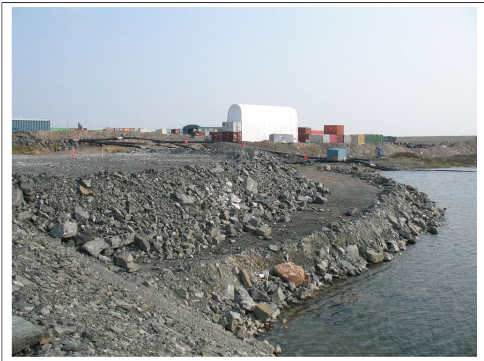
Photo #2 Whale Tail Dike, East abutment upstream thermal berm
