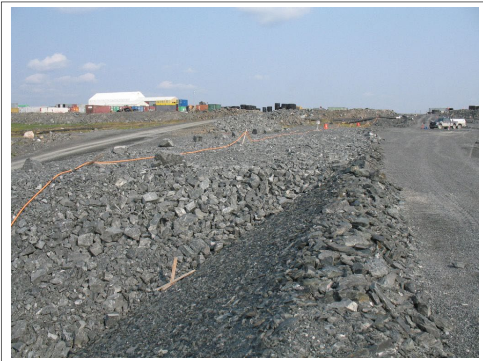
Photo #3 Whale Tail Dike, East abutment downstream thermal berm
