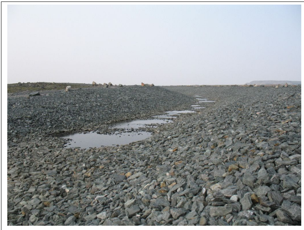
Photo #10 South Whale Tail Channel. Flow daylights in depressions
