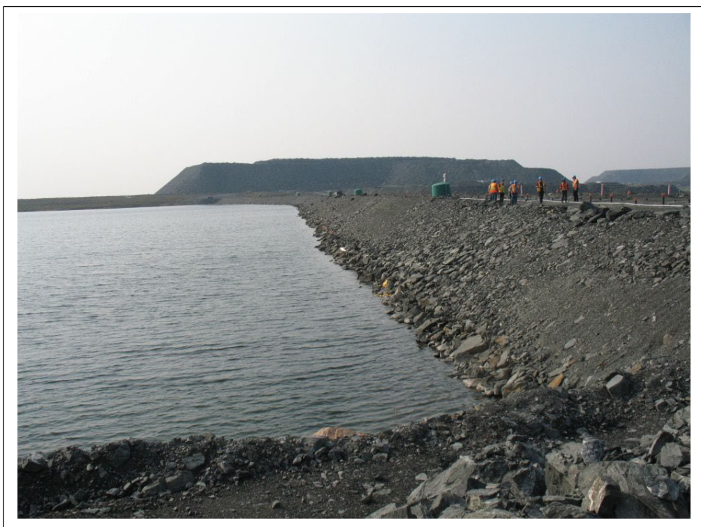
Photo #4 Whale Tail Dike, upstream face. Little if any wave damage.
