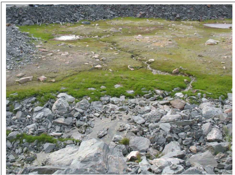
Photo #22 East Dike. Seepage and uplift? area noted in DSR
