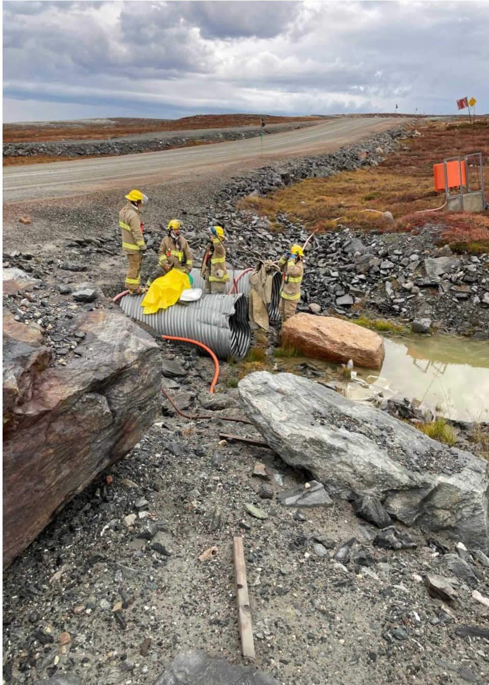
Figure 4 ERT members installing a culvert block
