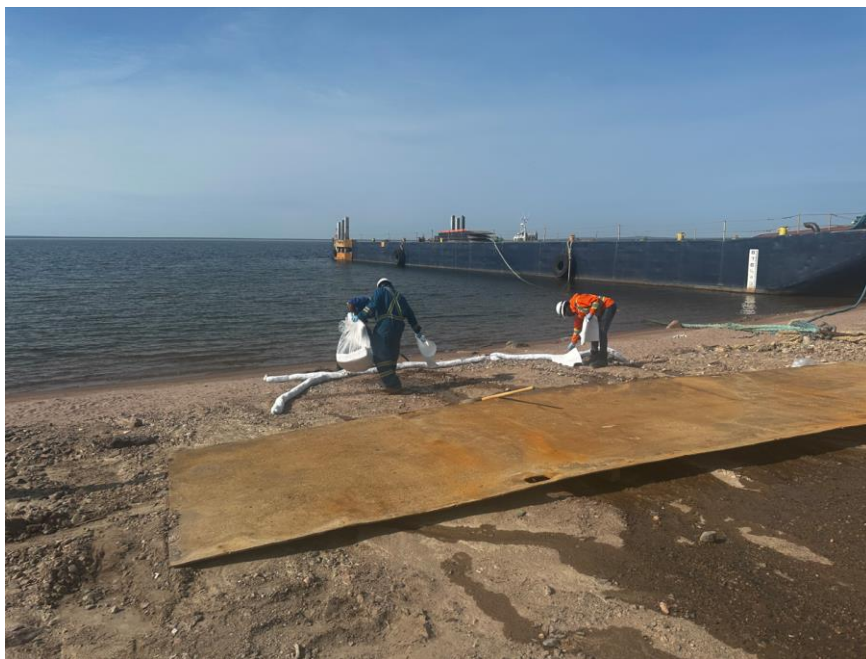
Figure 2 Utilizing spill booms and spill pad to control the flow.
