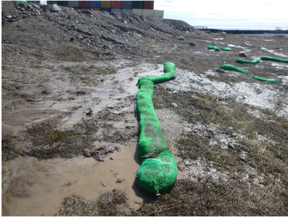
Figure 6. Additional turbidity controls installed to control water bypassing Ditch 2 and Splash Pad 2 (2024-06-15)
