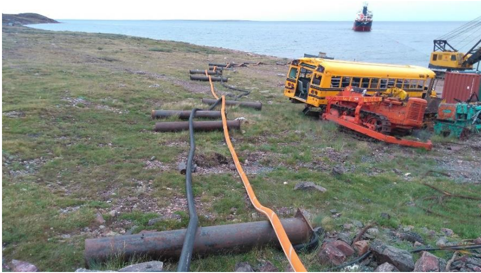
Photo 1. Diesel Transfer - Connection between shipper transfer hoses and Agnico Eagle permanent pipeline
