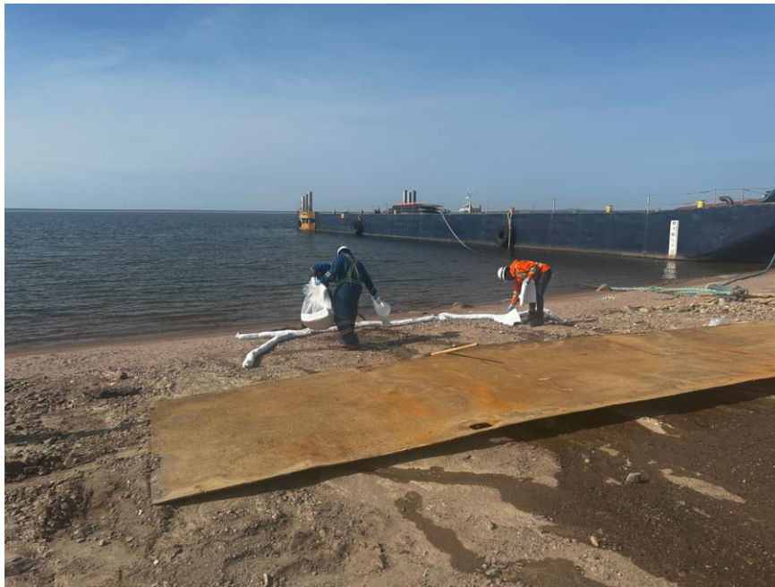
Figure 2 Utilizing spill booms and spill pad to control the flow.
