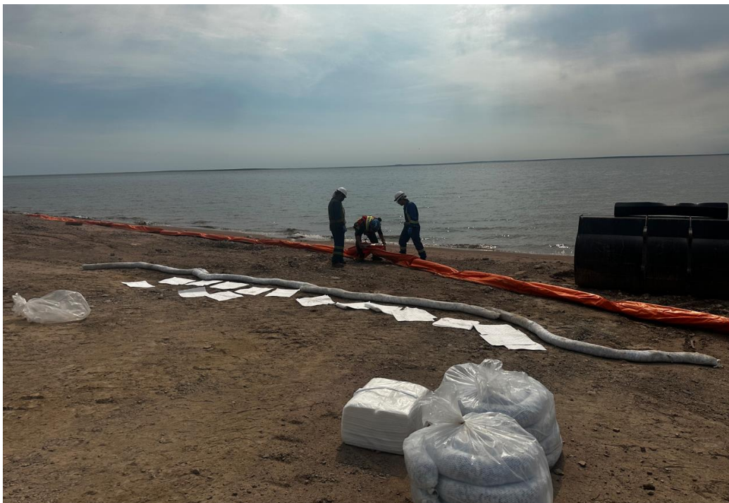
Figure 4 Assembling sections of the marine barrier prior to deployment.
