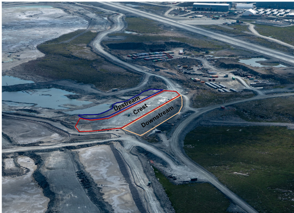
Figure 3-10: Aerial View of Saddle Dam 3
