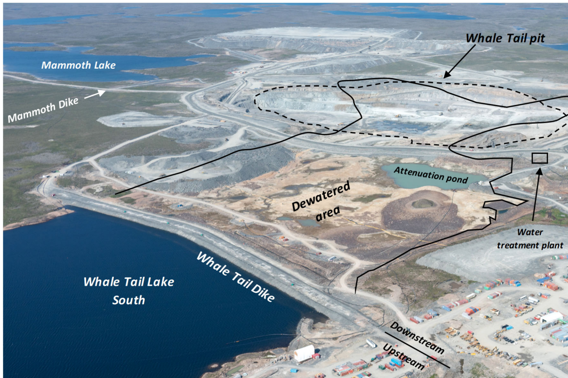
Figure 3-1 : Aerial View of Whale Tail Dike
