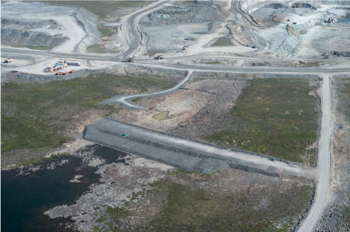
Figure 3-3 : Aerial View of Mammoth Dike
