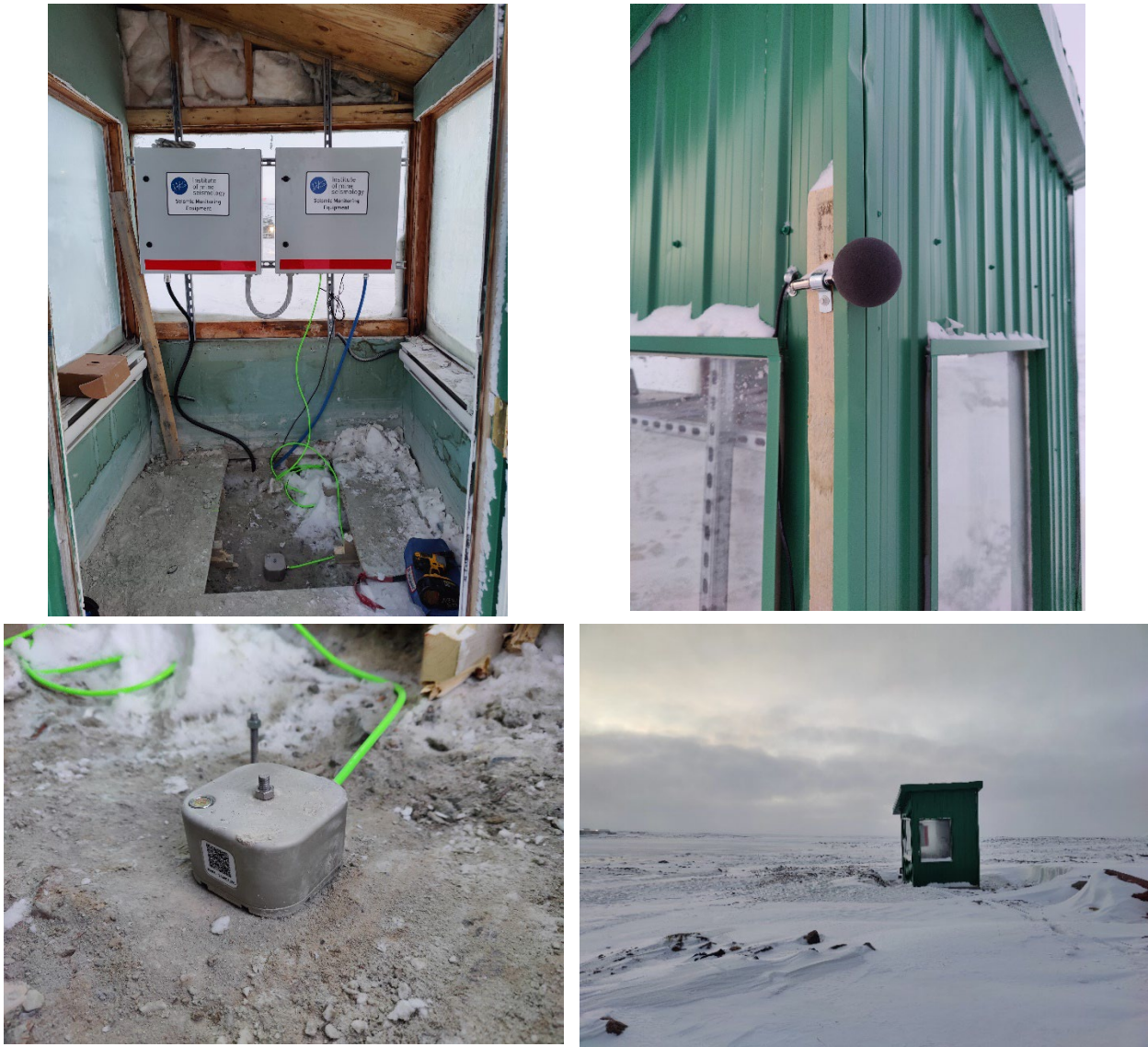
Figure 12 : Permanent blast monitoring installation
