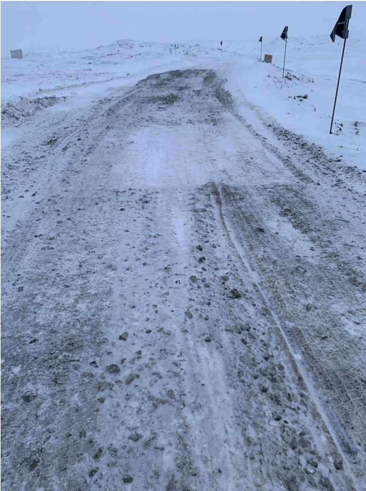
Photo 2: Final Cleanup (South)
