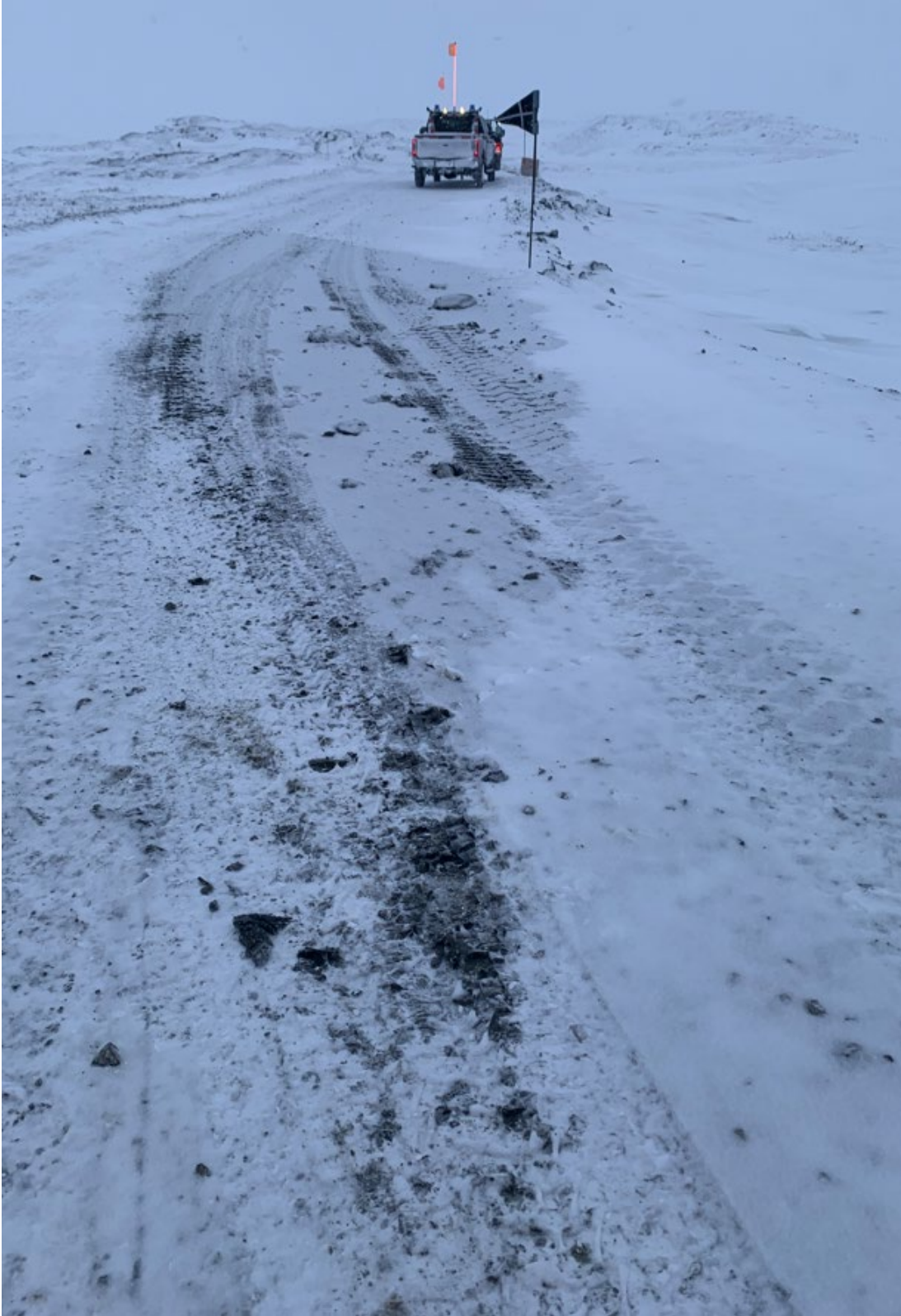
Photo 1: Frozen spill on gravel track (South)
