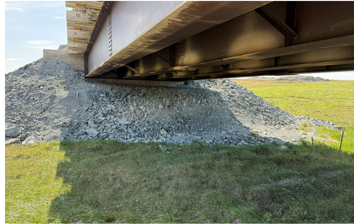
Photo 30: Doris-Madrid Road bridge 2/3 abutment inspection
