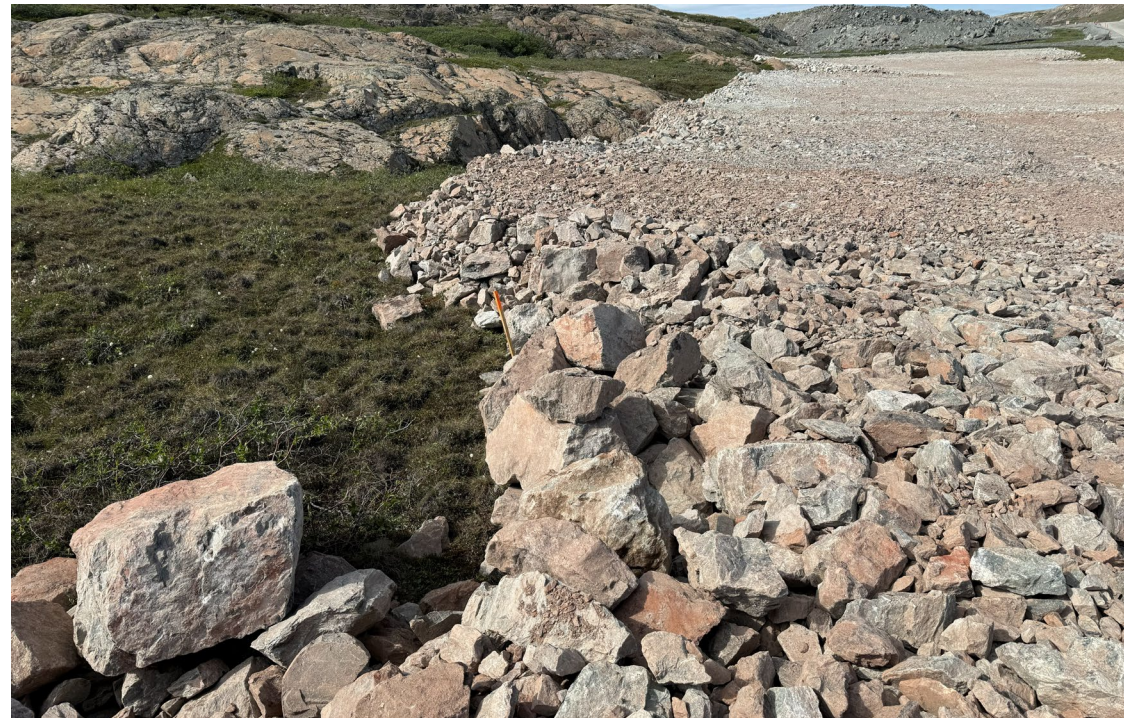
Photo 21: New laydown and Sewage Treatment Plant pad under construction
