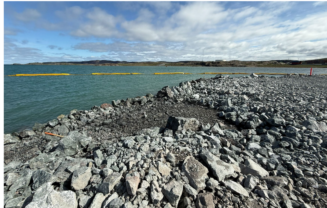
Photo 3: Roberts Bay Jetty, exposed geogrid for inspection (covered following inspection)
