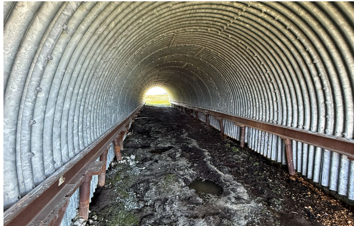
Photo 29: Doris-Madrid Road culvert inspection
