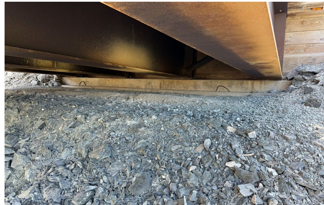
Photo 32: Doris-Madrid Road bridge 2/3 abutment inspection
