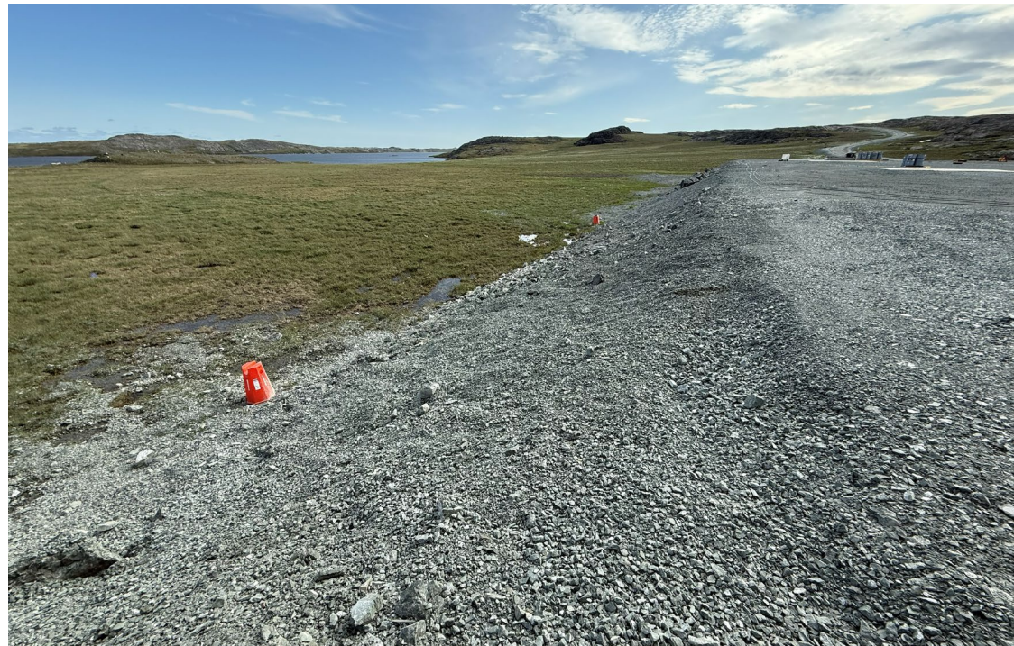
Photo 23: Helicopter pad downstream slope
