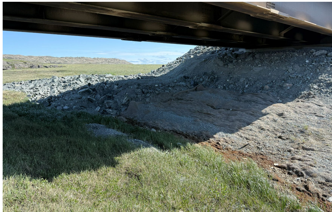
Photo 31: Doris-Madrid Road bridge 2/3 abutment inspection
