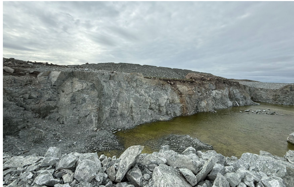
Photo 37: Madrid North Sump 1 west wall
