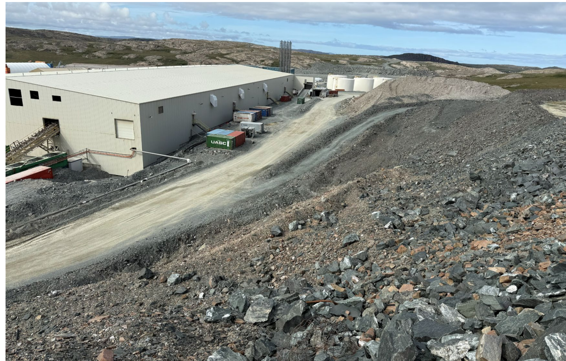
Photo 17: Pad T waste rock slope
