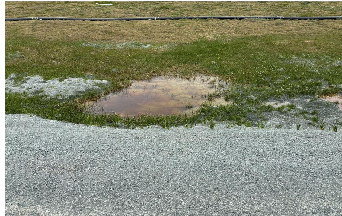
Photo 28: Water accumulation on the west side of the airstrip
