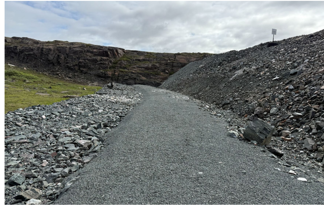
Photo 18: Doris Diversion Berm – upstream end, looking east
