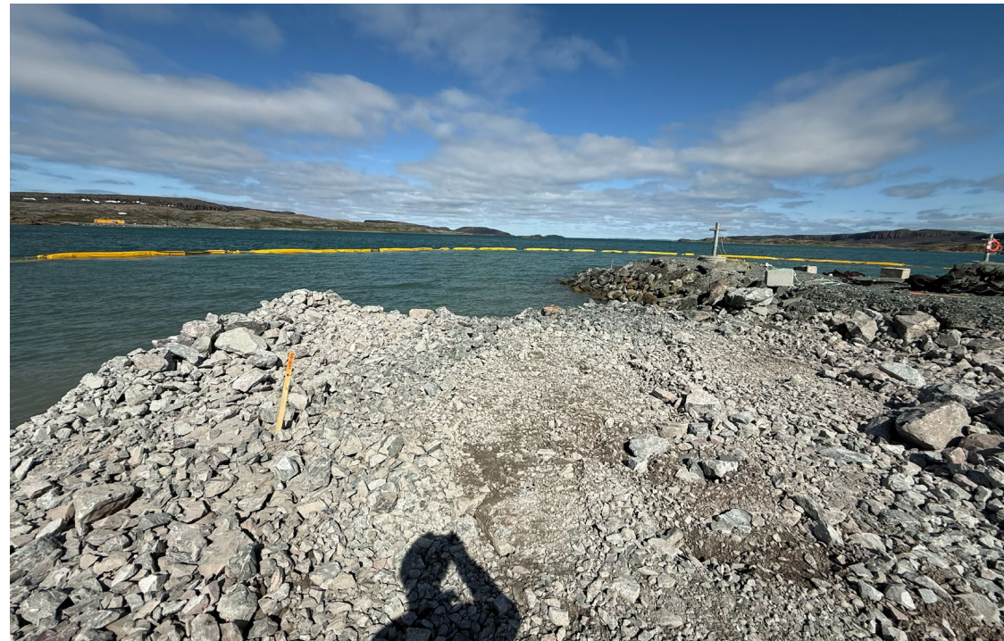
Photo 1: Roberts Bay Jetty overview
