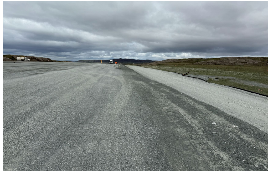
Photo 25: Airstrip east shoulder, looking north
