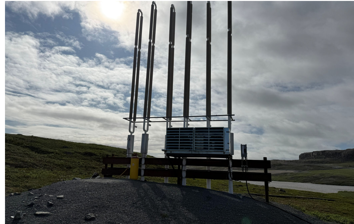
Photo 6: North Dam South Thermosyphon Bank
