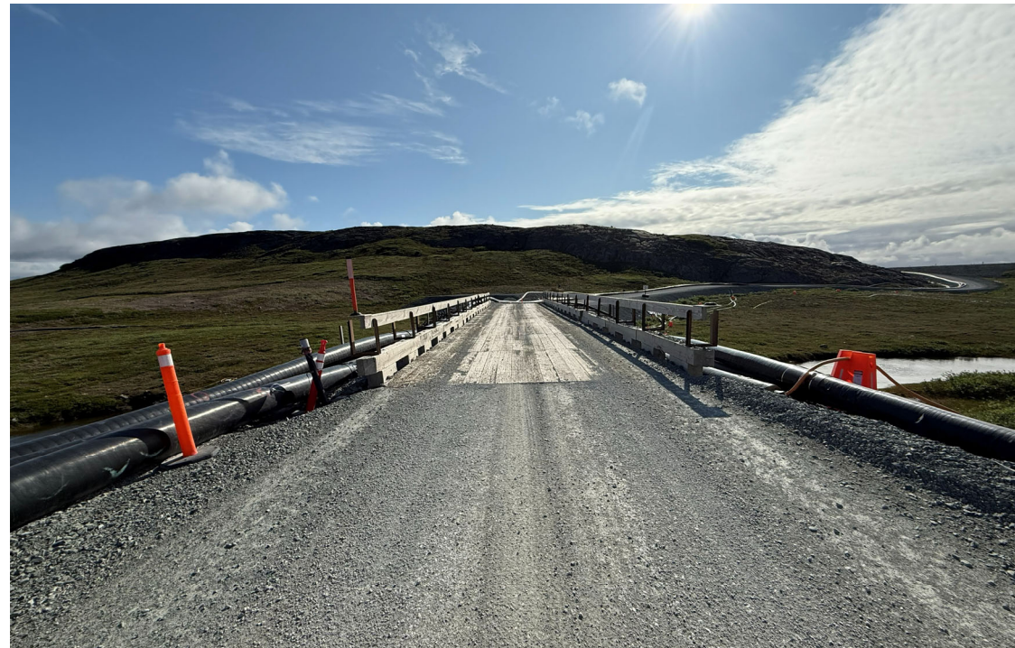
Photo 29: Doris Bridge Overview
