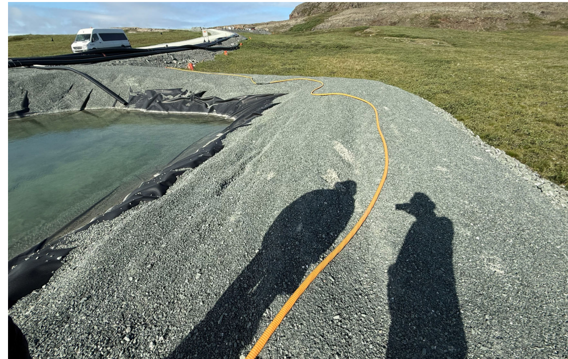
Photo 28: Western Emergency Dump Catch Basin Slope
