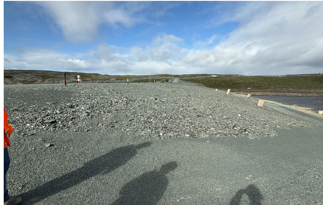
Photo 2: North Dam Upstream Face
