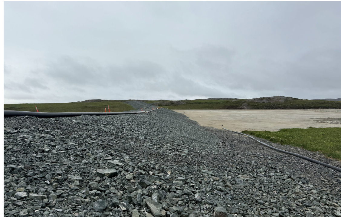
Photo 11: North Dam Upstream Face
