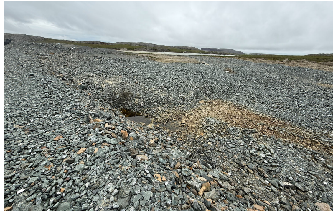
Photo 22: Interim Dike Interim Dike Water Elevation Control Channel
