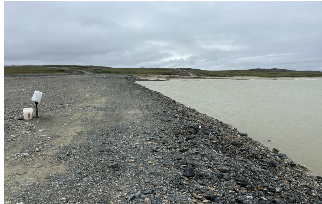
Photo 20: Interim Dike Upstream Face
