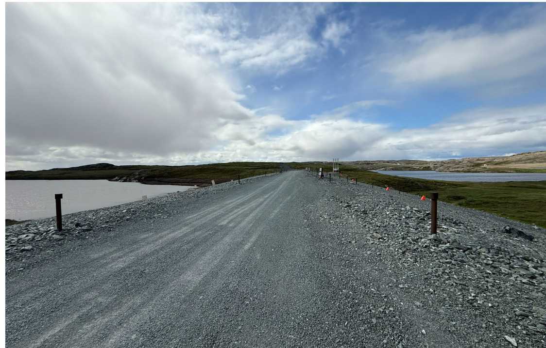
Photo 1: North Dam Crest Overview
