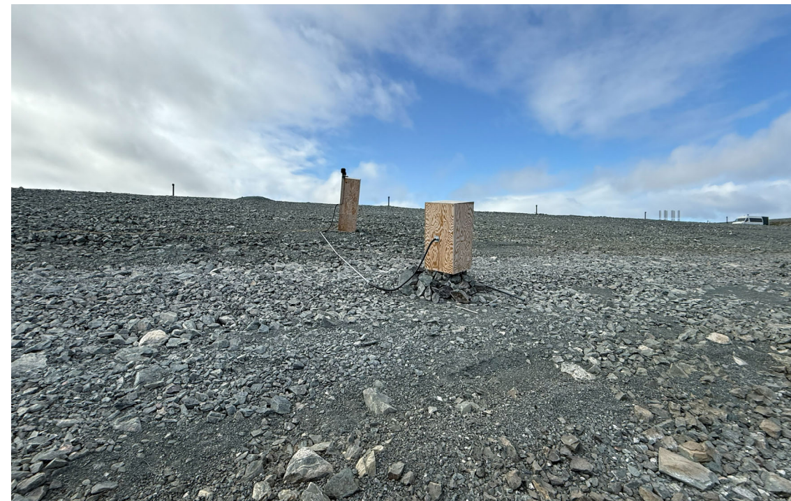
Photo 8: North Dam Instrumentation Inspection
