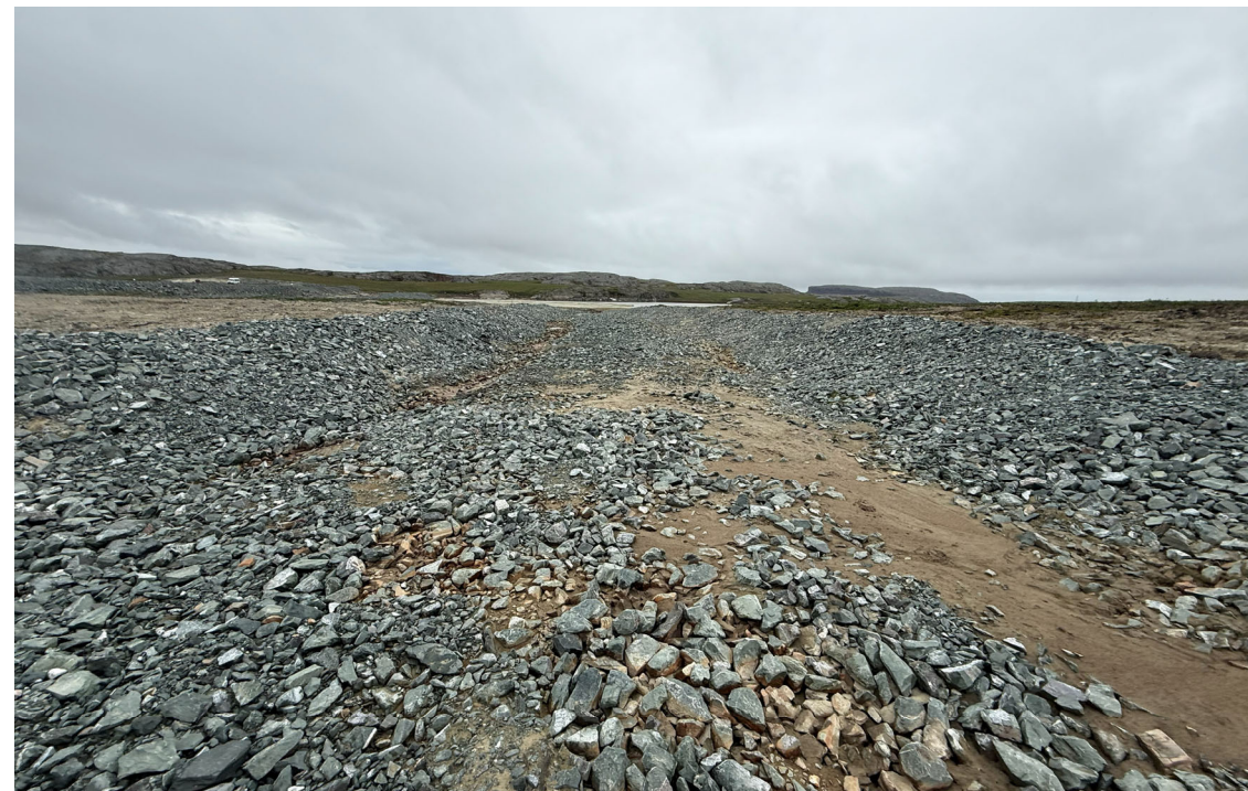
Photo 24: Interim Dike Water Elevation Control Channel Base Near Invert
