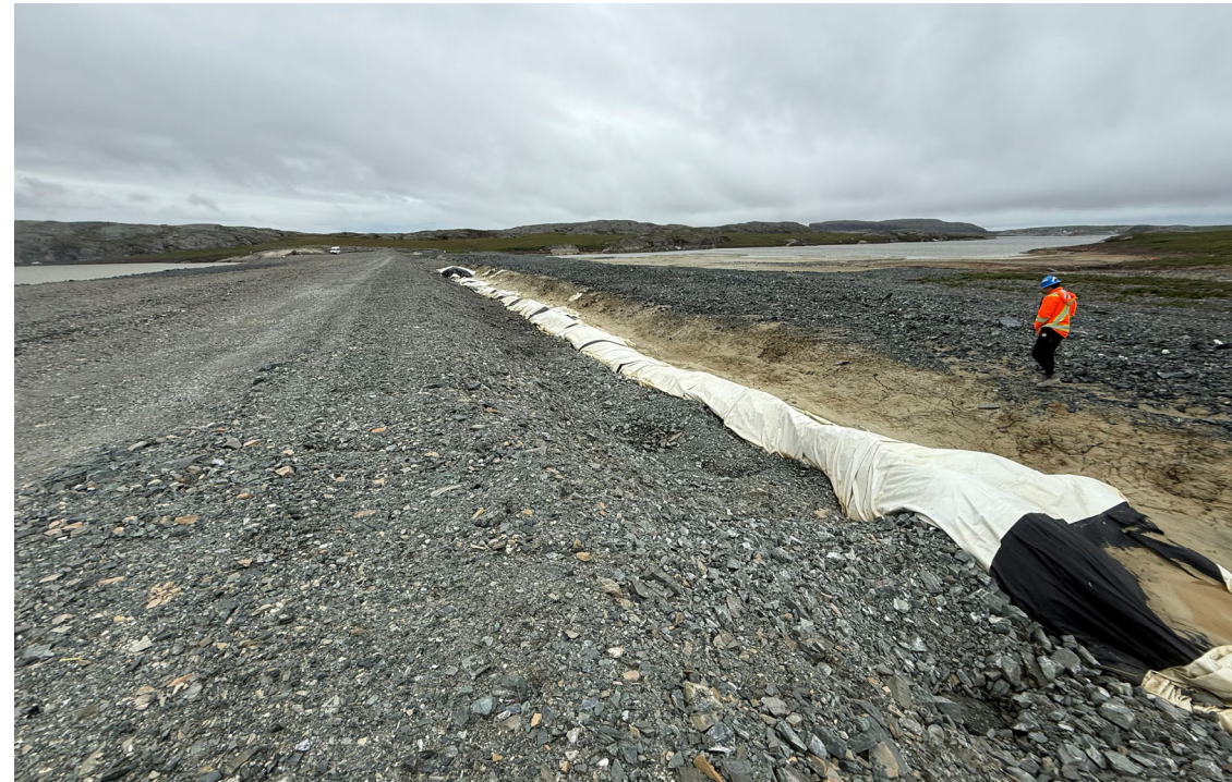
Photo 18: Interim Dike Overview and Former Aquadam Location (Looking West).
