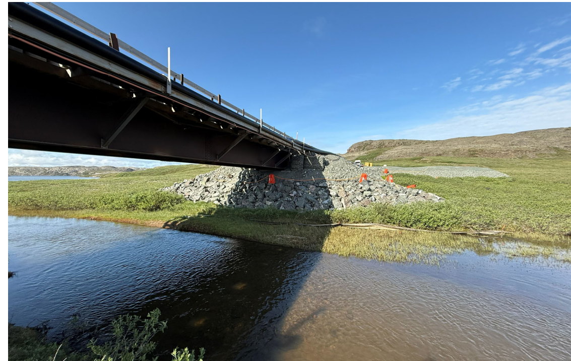
Photo 32: : Doris Bridge Overview Below the Deck
