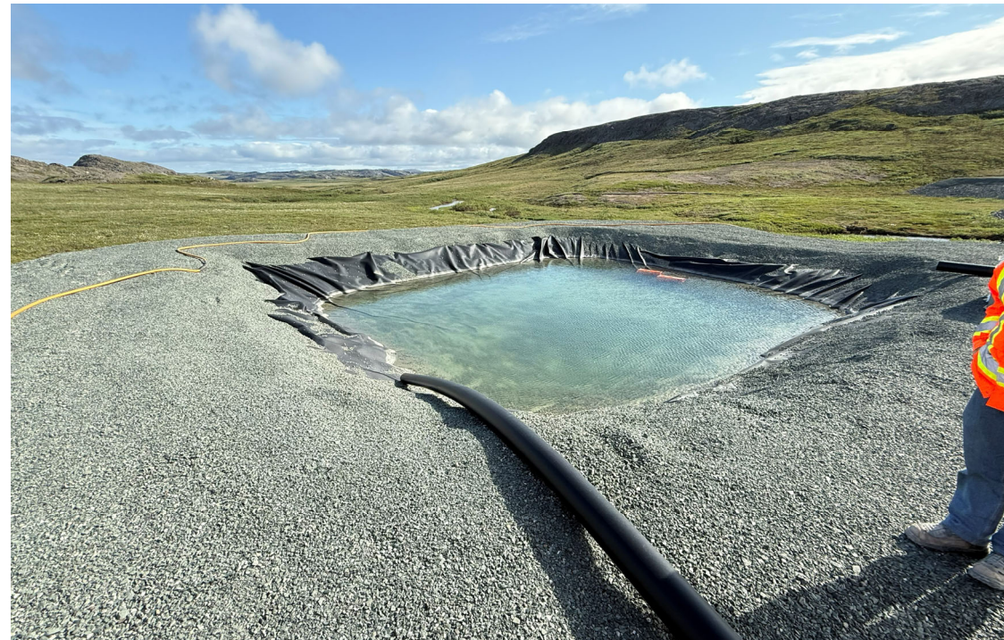
Photo 27: Western Emergency Dump Catch Basin
