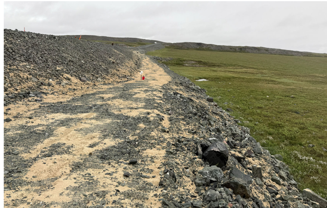
Photo 12: South Dam Downstream Toe Berm
