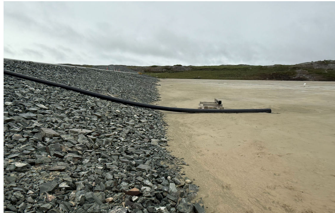
Photo 15: South Dam Upstream Face
