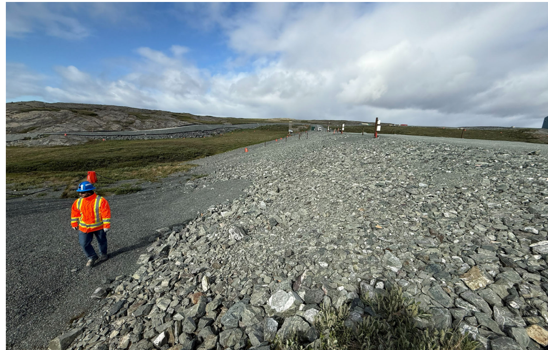
Photo 3: North Dam Downstream Face
