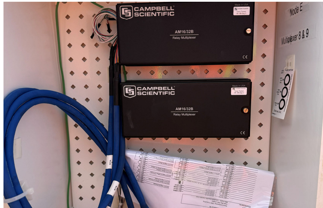
Photo 7: North Dam Instrumentation Inspection
