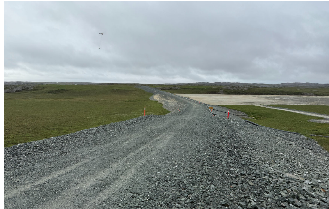
Photo 10: South Dam Crest Overview
