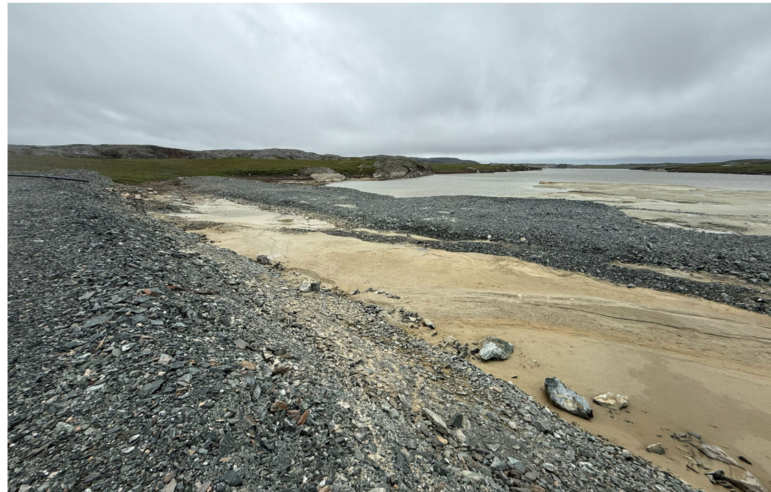
Photo 17: Interim Dike Downstream Slope Overview
