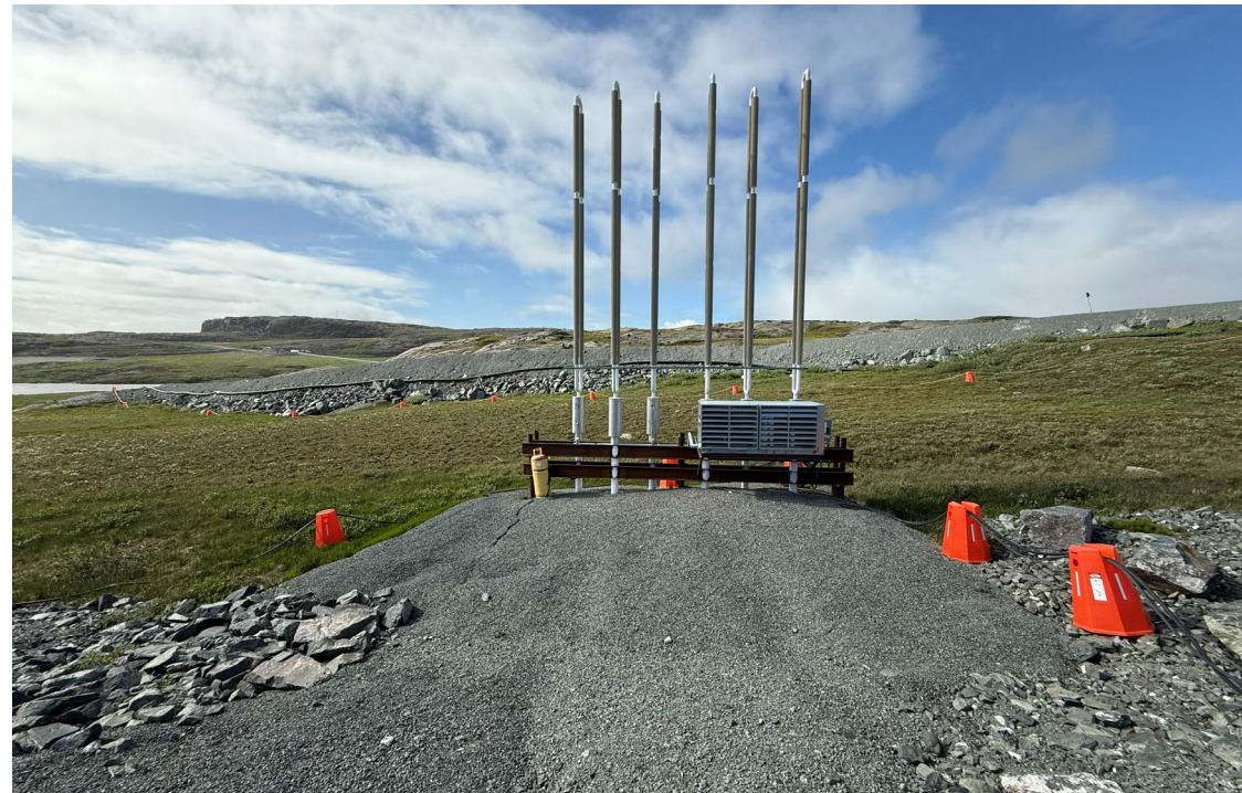
Photo 5: North Dam North Thermosyphon Bank
