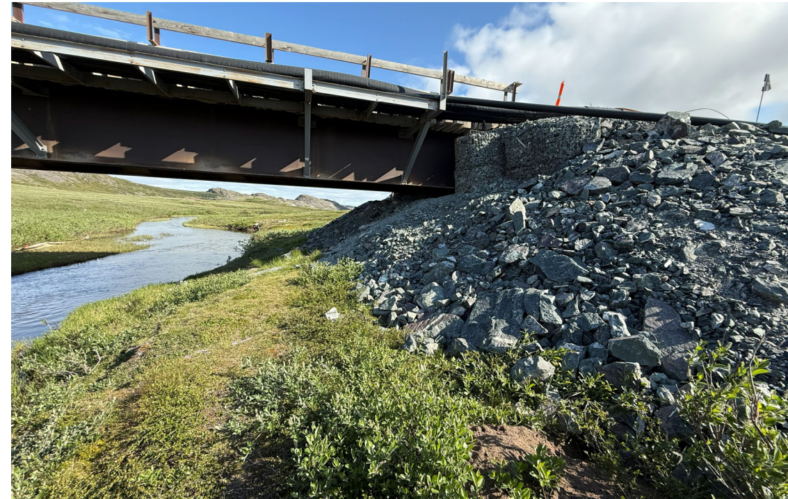
Photo 30: Doris Bridge Abutment and Gabion Inspection
