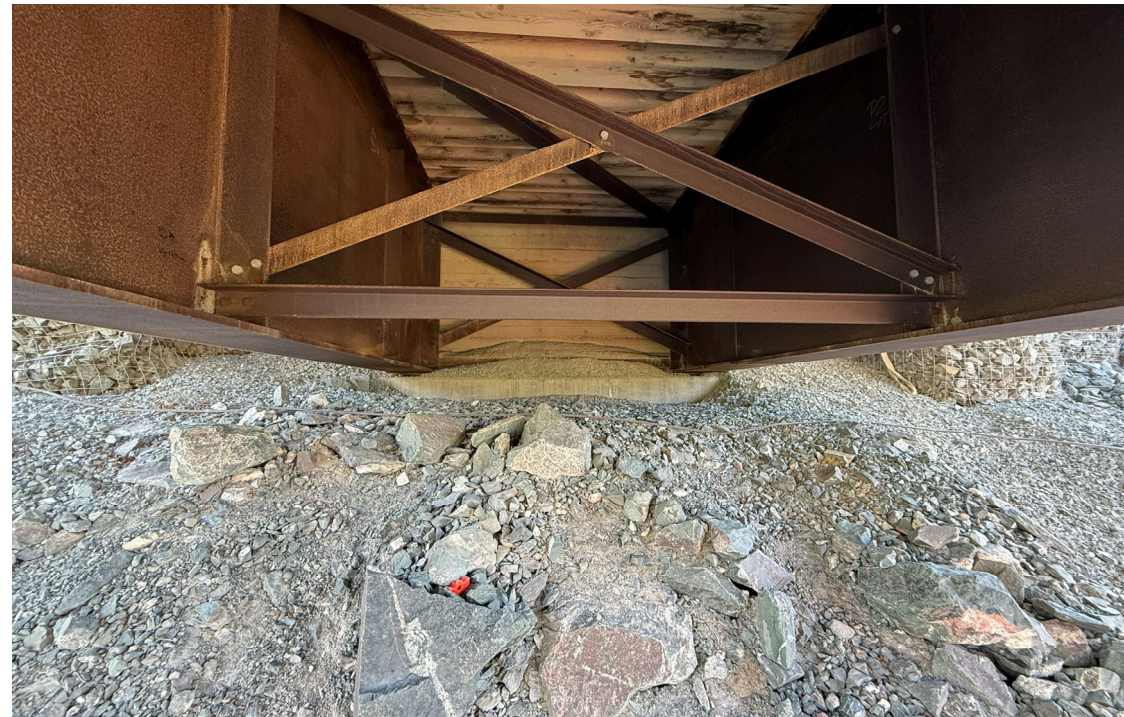
Photo 31: Doris Bridge Inspection
