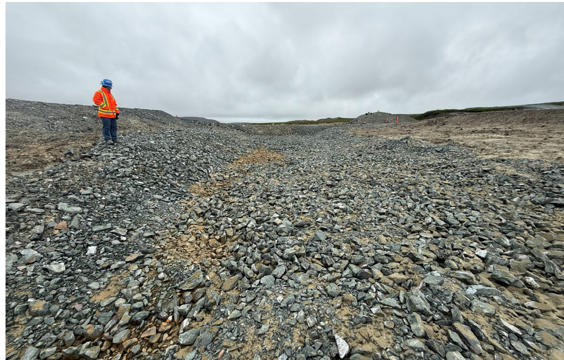
Photo 21: Interim Dike Water Elevation Control Channel
