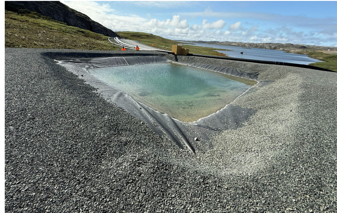
Photo 26: Eastern Emergency Dump Catch Basin
