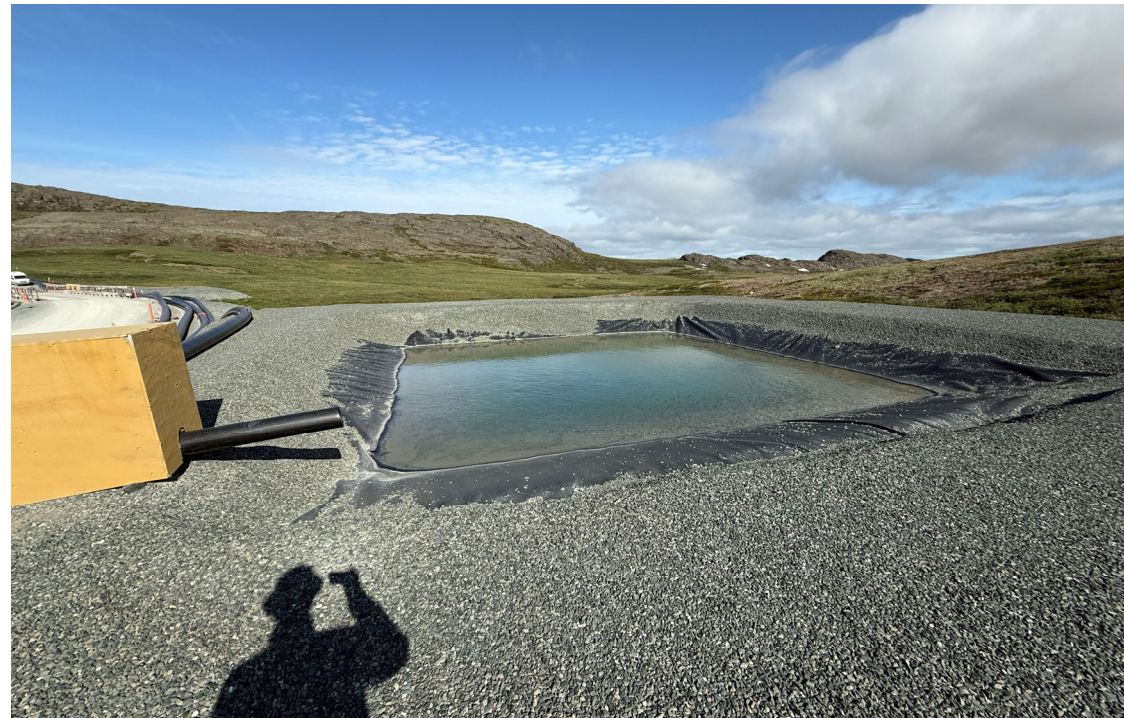
Photo 25: Eastern Emergency Dump Catch Basin
