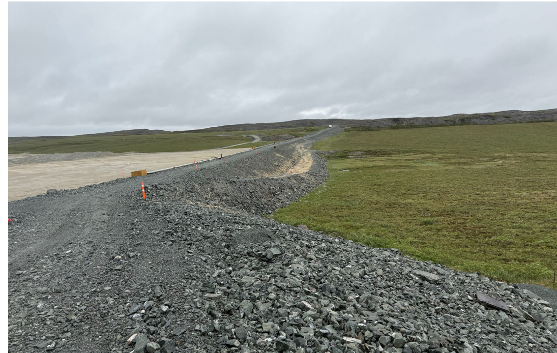
Photo 14: South Dam Downstream Toe Berm
