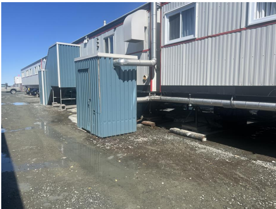
Photo 2: Spill location post remediation
