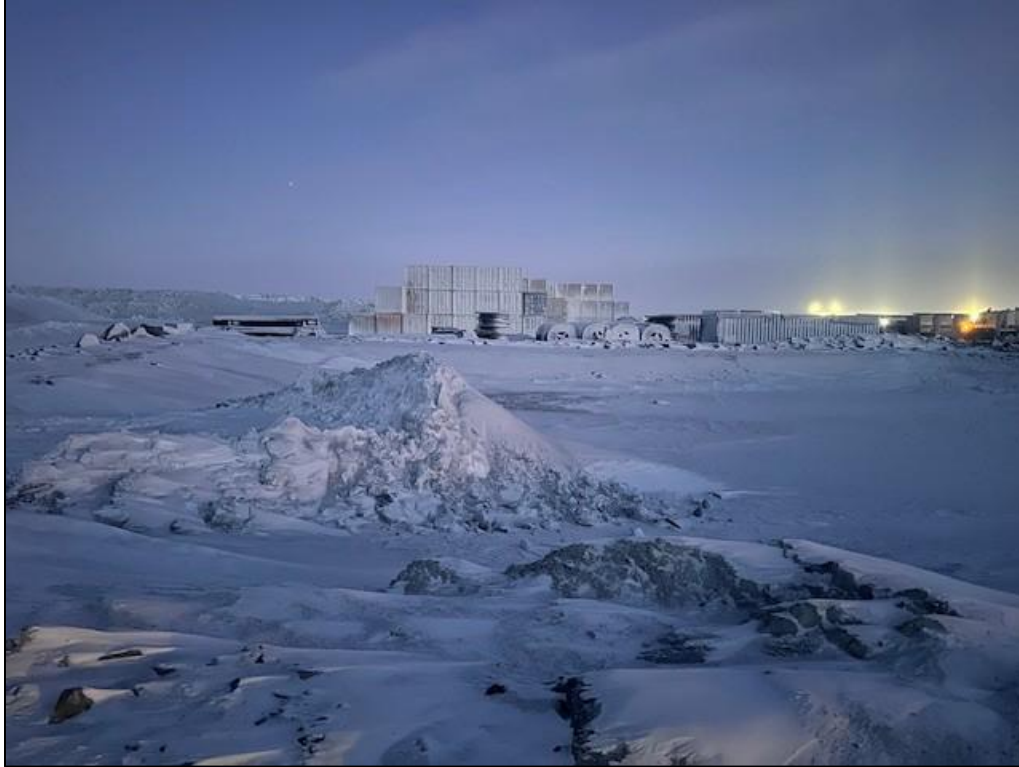
Photo 4: Material collected and placed at the contaminated Snow Cell
