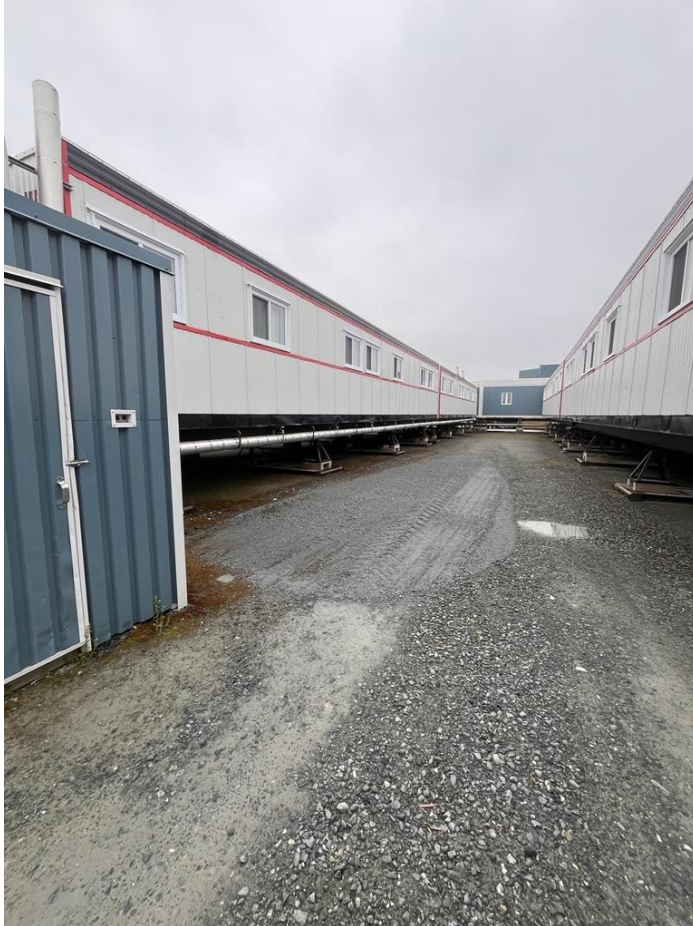
Photo 2: Spill location post remediation
