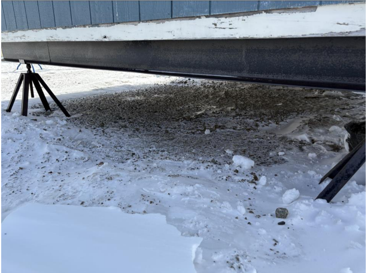
Photo 2: Spill location post remediation
