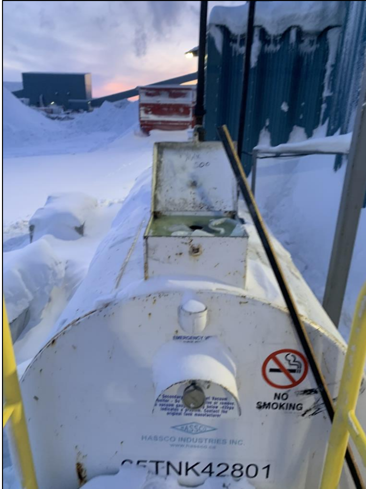
Photo 1: Diesel spill location, at the incinerator laydown.
