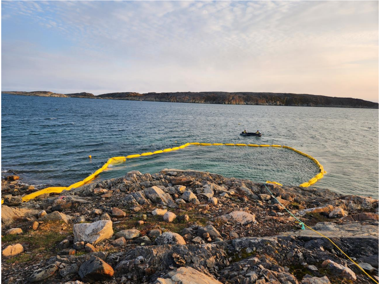
Photo 2: Turbidity curtains installed before resuming the drilling operation.
