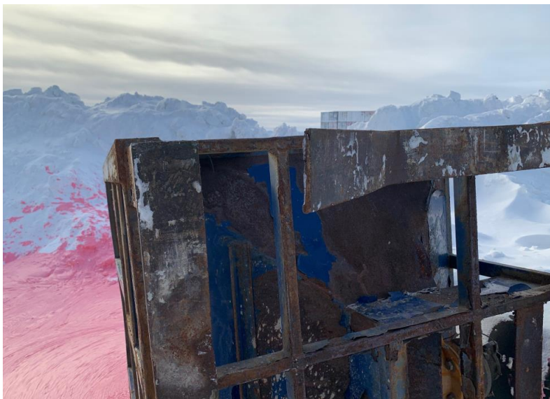
Photo 2: Broken base plate on the bin.
