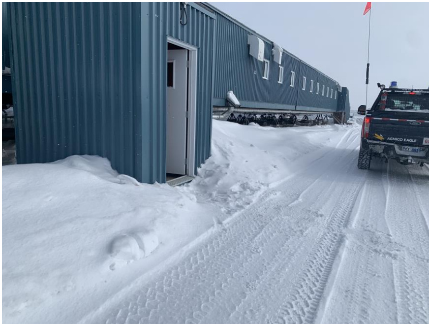
Photo 2: Spill location post remediation
