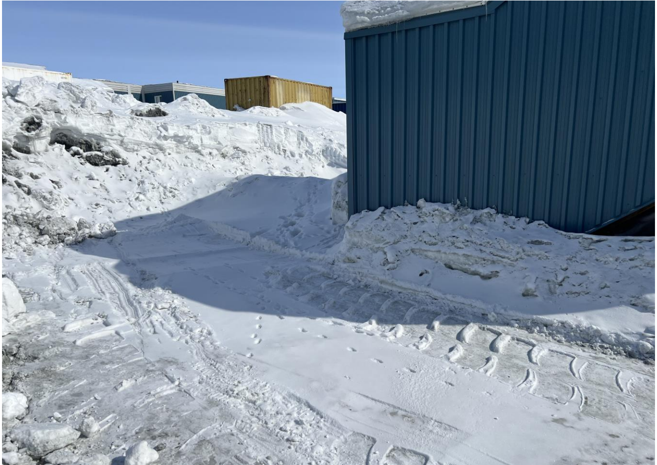
Photo 3: Sewage spill location post excavation of accessible contaminated material
