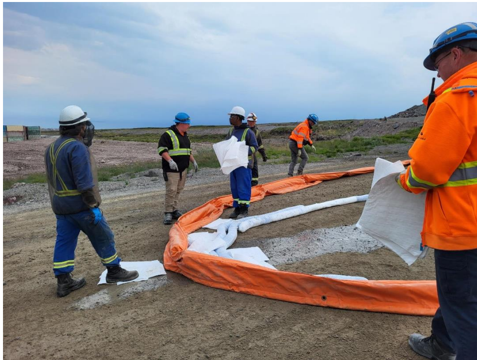
Tying sections of barrier before deployment.
