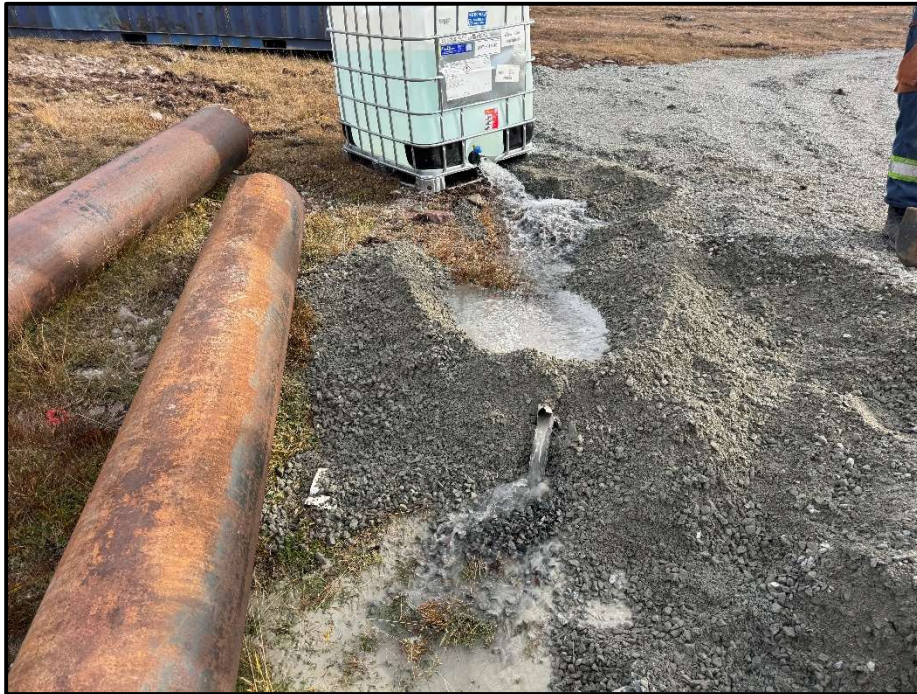
Photograph 3: View of simulated fluid release with constructed inverted weir.
