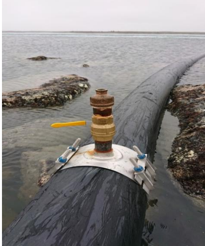
Photo 5. ST-MDMER-7 FDP before dismantling
