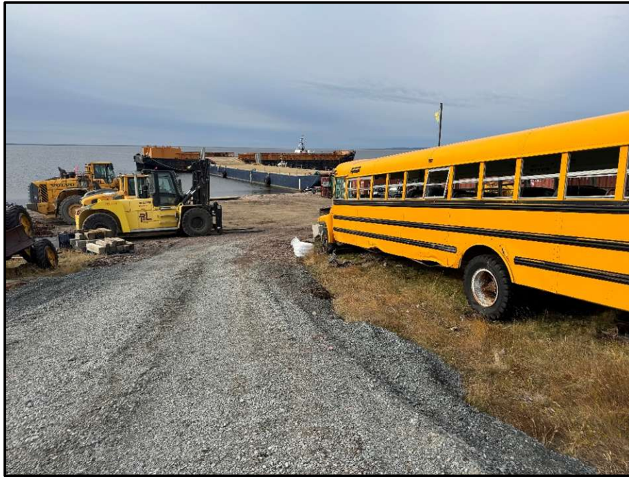
Photograph 1: View of access facing south towards Baker Lake
