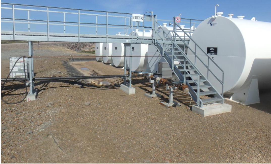
Photo 2. Jet-A Transfer - Connection between shipper transfer hoses and Agnico Eagle permanent pipeline
