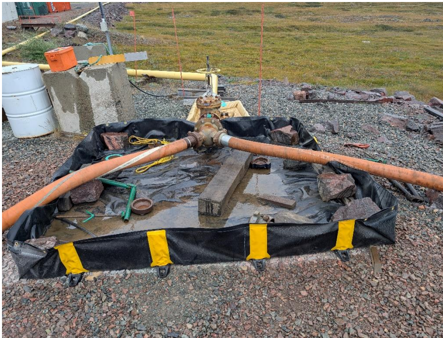
Photo 1. Portable Containment pool at the connection of the ship's conduit to the OHF manifold
