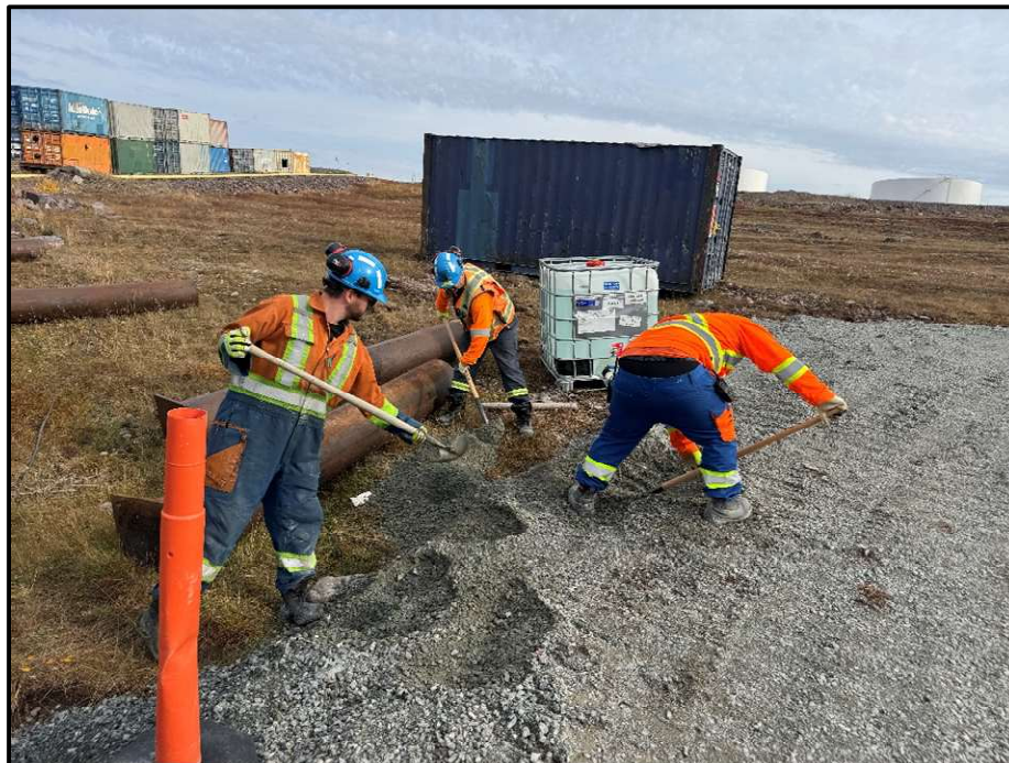
Photograph 4: Construction of inverted weir
