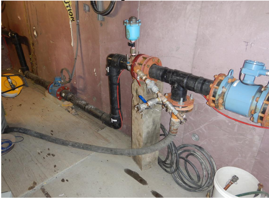
Photo 2. FDP East Dike Discharge Meadowbank
