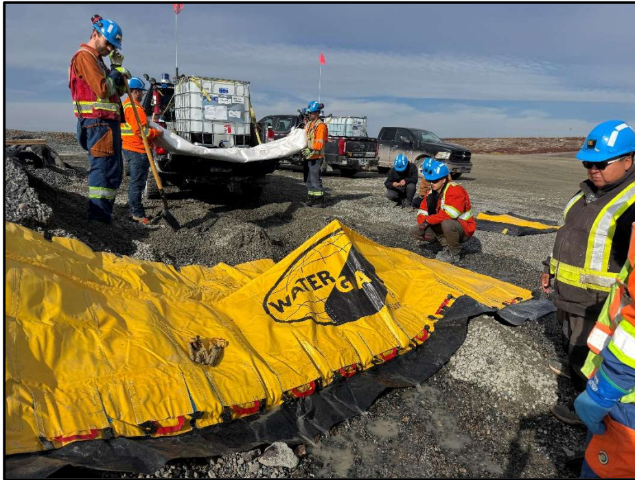
Photograph 5: Deployment of a watergate.
